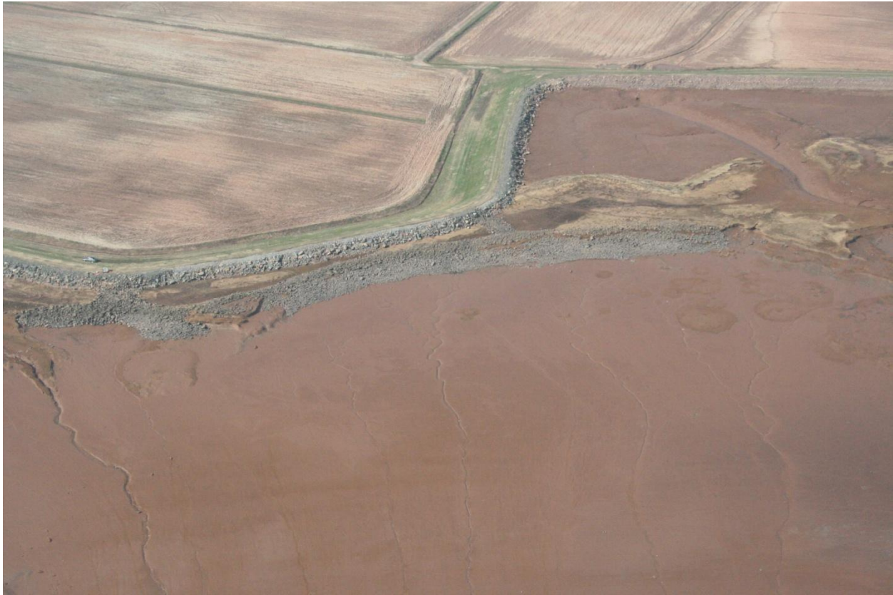
Figure 13: Coastal erosion is a constant pressure on the dykes. Above is a picture of the east facing dykes at extreme low tide. Top right corner: remnants of the salt marsh. In the middle: rock facing on the dykes and breakwater. Both have been weakened by the constant tidal pressure.
