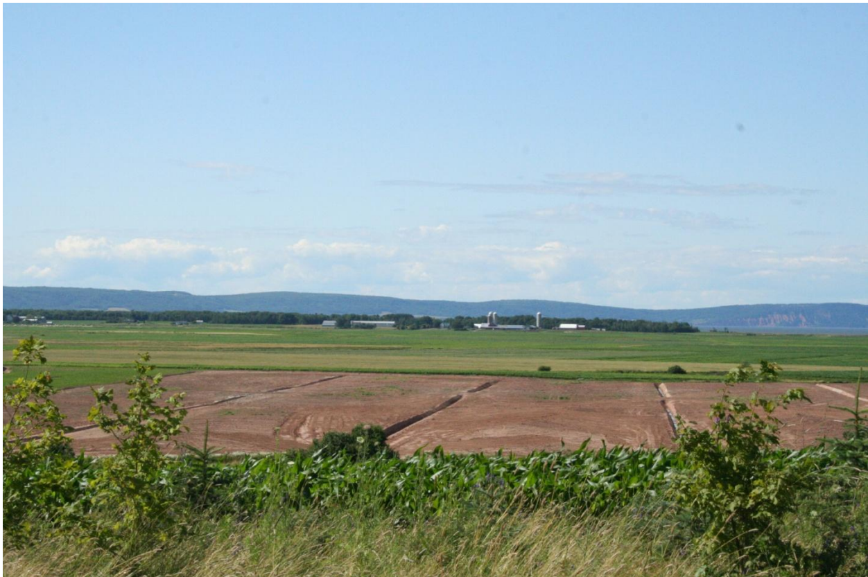
Figure 15: Drainage work on a field in Hortonville.
