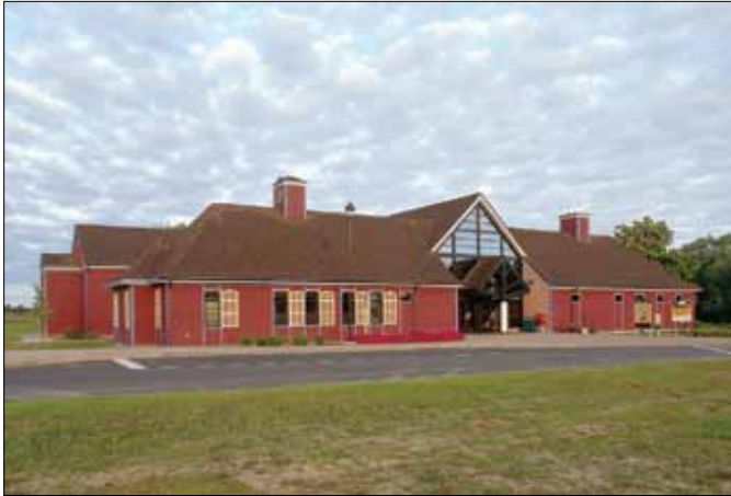
5-5 The visitor reception and interpretation centre at Grand-Pré National Historic Site of Canada, constructed in 2003, is a key feature of the tourism management strategy for the nominated property.
